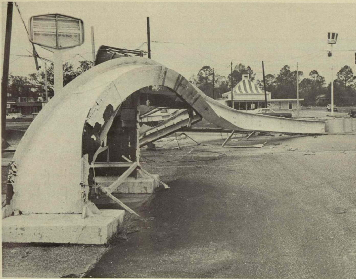
Steel I-beam support was no match for the brute strength of Hurricane Frederic.
